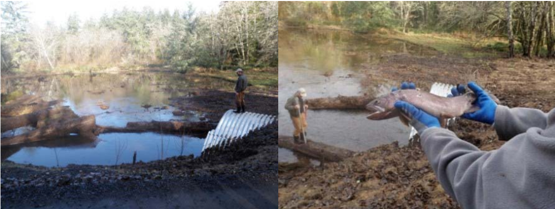
New culvert and RCG scrape down area (left); wild cutthroat found at site (right).
