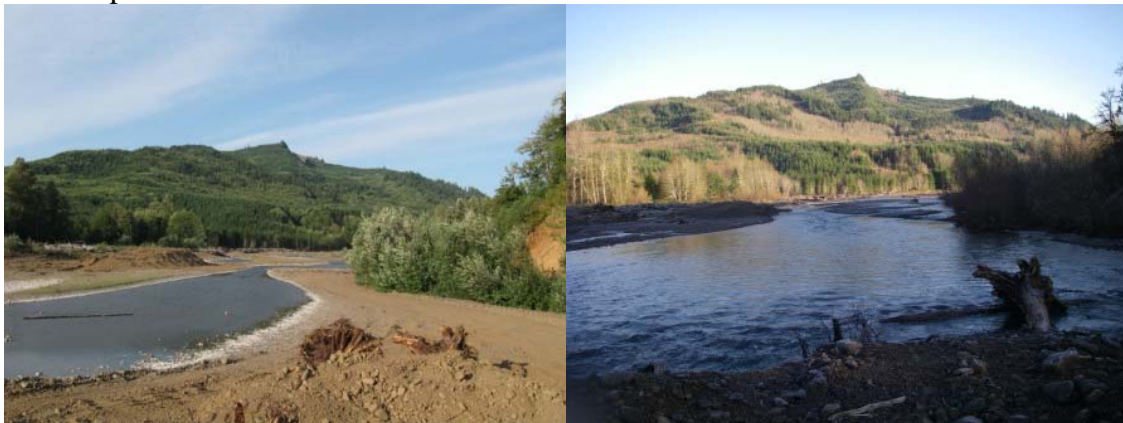
Newly buried ELJ structures at summer flow (left); the return of winter flow (right).
